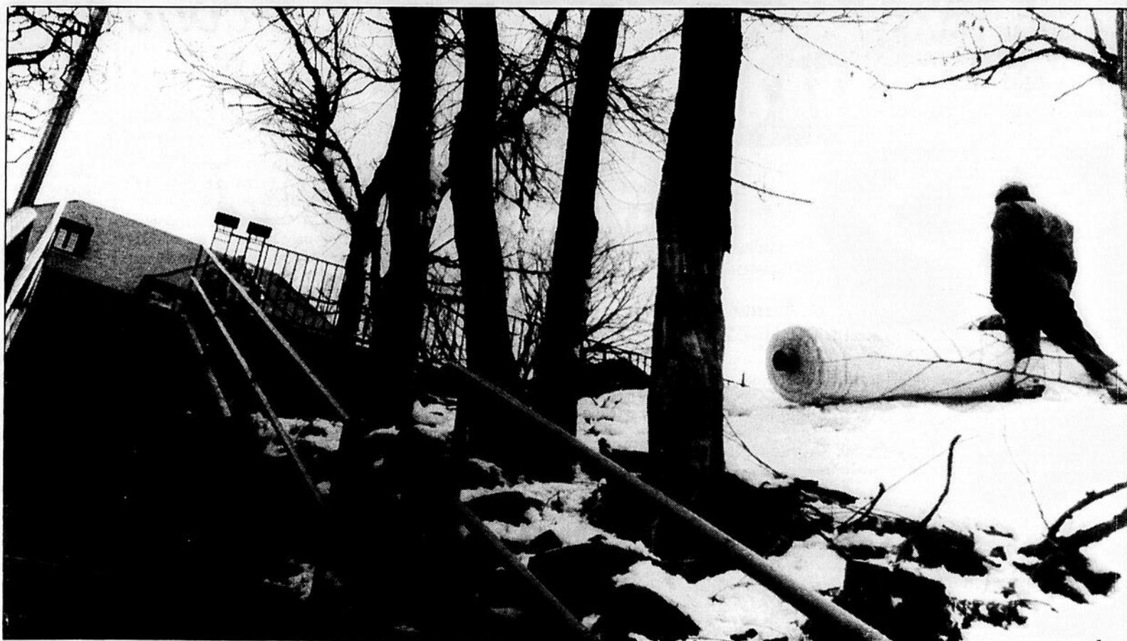
Aménagement Côté Jardin contractors unroll the mesh that will stabilize the embankment of 36 Sunnyside Ave. The public steps
