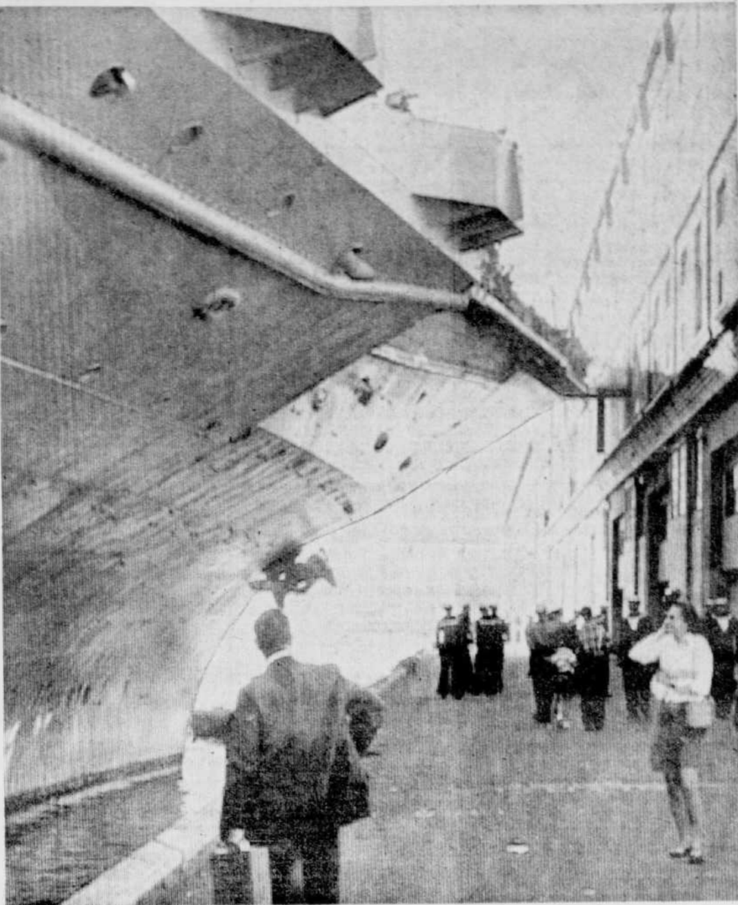
DEAD AHEAD — Bystanders on the Halifax waterfront were unaware that the 40,000-ton American aircraft carrier Essex was about to pay an unexpected visit on the immigration building. The flight deck of the ship is shown just as it struck the second floor of the building, making a shambles of a medical officer's office. (CP Wirephoto)
