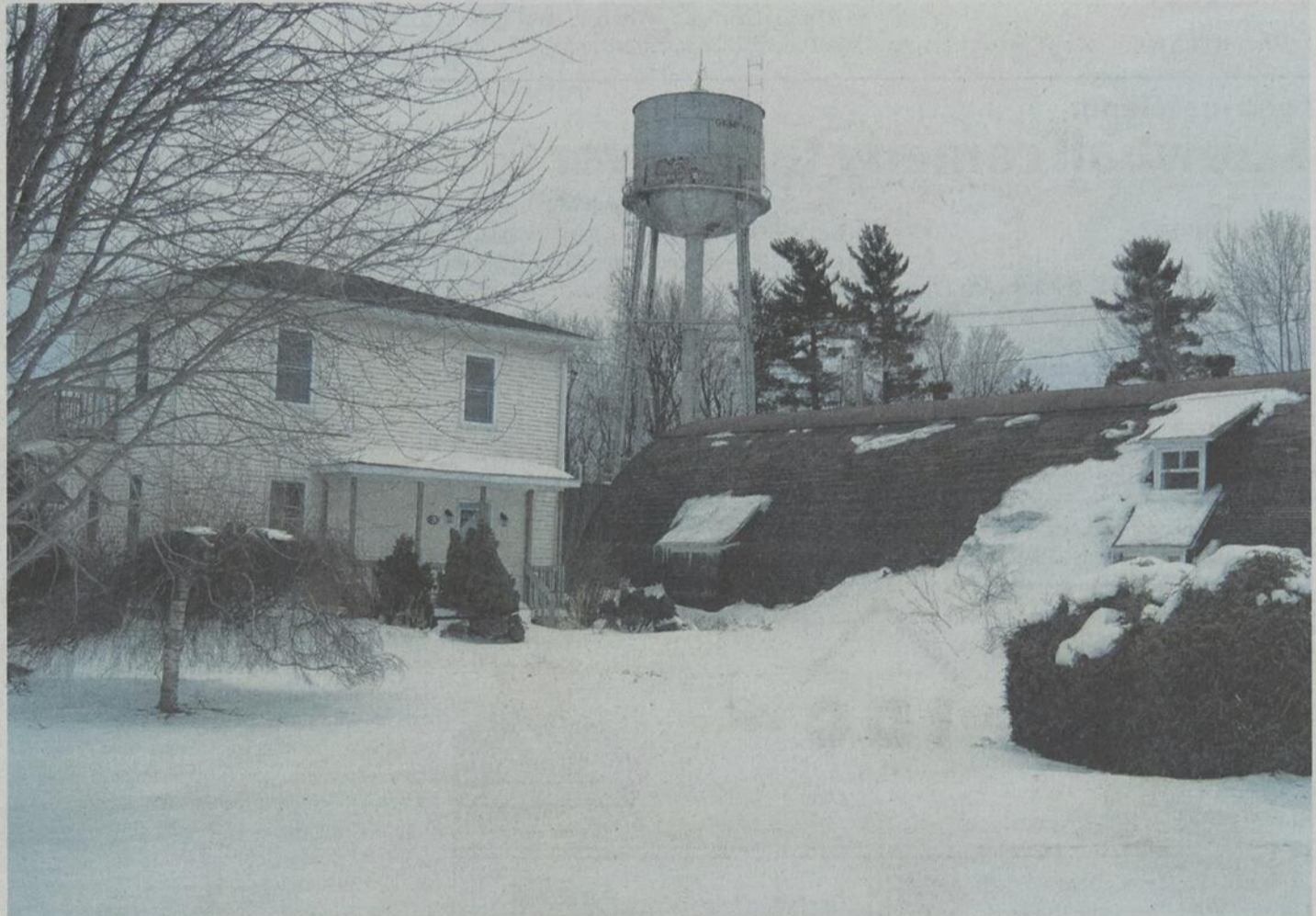
Once the Municipality of Ormstown owns 3 Gale Street it will proceed to demolish the residence there. (TC M dia-Archives)
