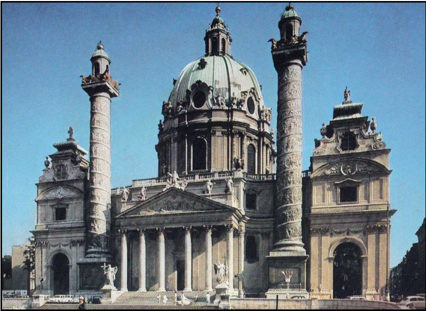
Figure 2.10: Saint Karl's Cathedral designed by Fischer von Erlach (1656–1723).
