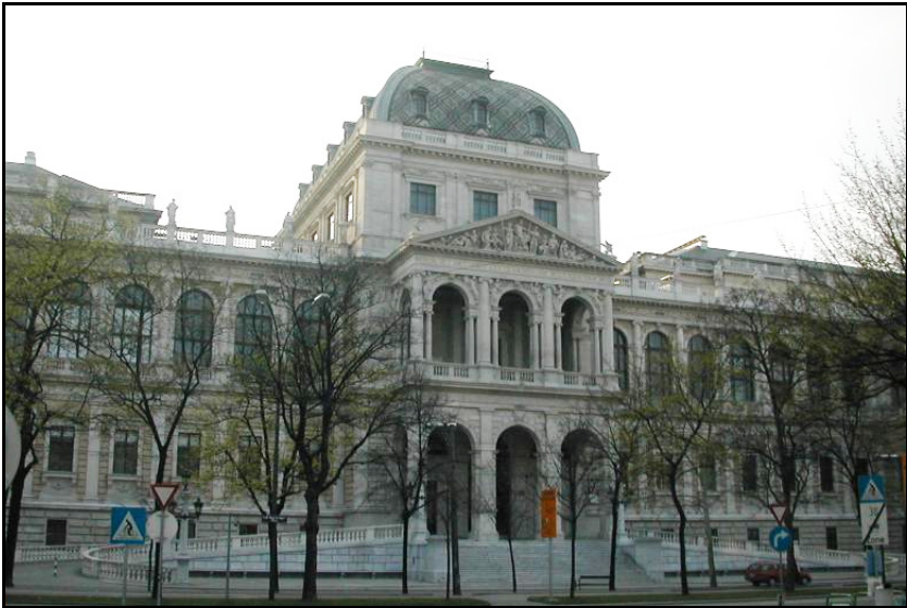
Figure 1.15: University of Vienna new building on Ringstraße.
