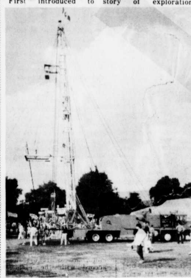
SERVICE RIG, with its towering 69-foot mast, is the centre of attraction of the OUR PETROLEUM CHALLENGE display, designed to take the story of Canada's petroleum industry to the public.
