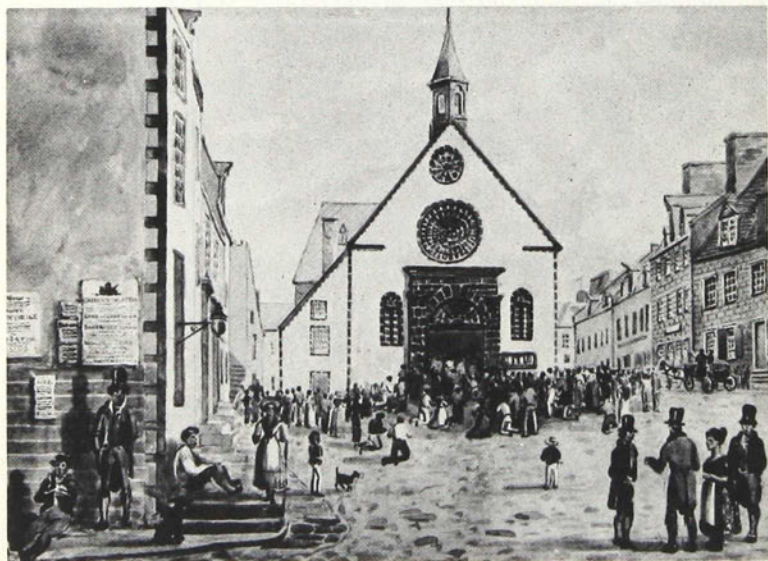
Fig. 8-A Place Royale in 1831. Notre-Dame des Victoires church with, on the left, the Marie-Anne Barbel house, built in 1754.
