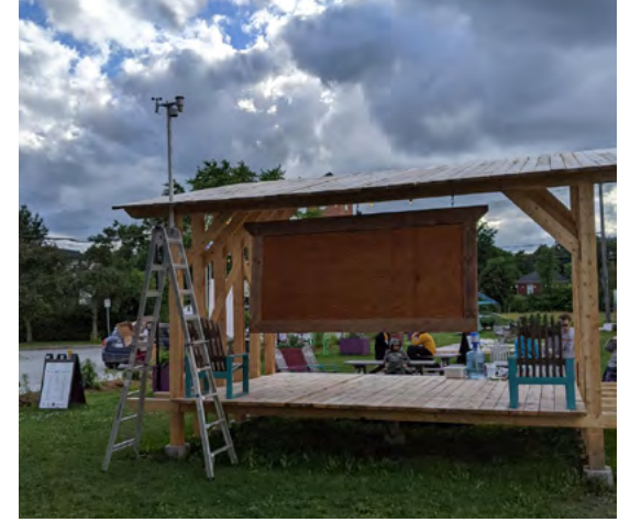
Installation de la station   Lennoxville
