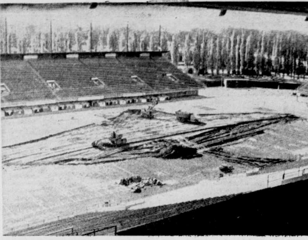
PREPARING THE FIELD—Workers using heavy construction equipment continue the nine-day facelifting job at Lansdowne Park preparing for the Dec. 2 Grey Cup game at Ottawa. They will strip the sod from the field and replace it with thicker turf. Work began Sunday. (CP Wirephoto)
