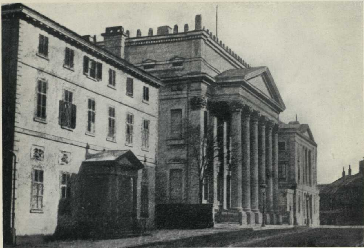
OLD BUILDING—BANK OF MONTREAL
