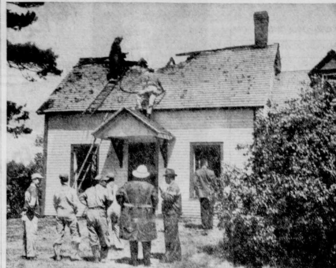
ST. ELIE FIRE — Seen above is the small home on the St. Elie road belonging to Jean Paul Quirion which suffered about $1,500 worth of damage yesterday when flames broke out in the upper floor of the frame building. The house was in the process of being renovated.
