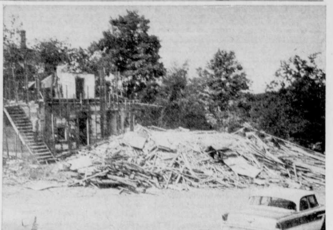
BILTRITE EXTENSION — The house, above, on William St., property of the American Biltrite Rubber Company adjoining the Jenckes St. plant, is being demolished to make way for a $4,000,000 extension which will add 300 additional male workers to the payroll. (Record photo by Gerry Lemay)
