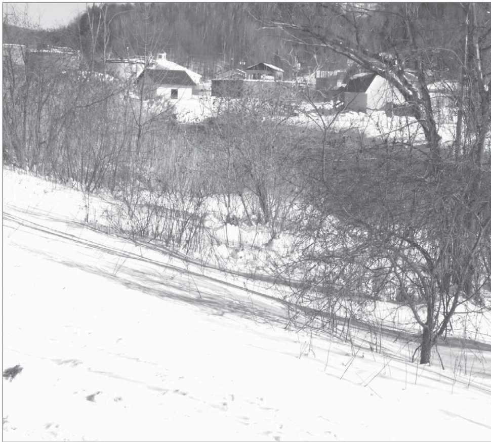
The Newport wastewater treatment plant sits on the Clyde River, which empties into Lake Memphremagog in Newport, Vermont and treats 15,000 gallons of leachate daily from the Vermont state landfill site at Coventry.
