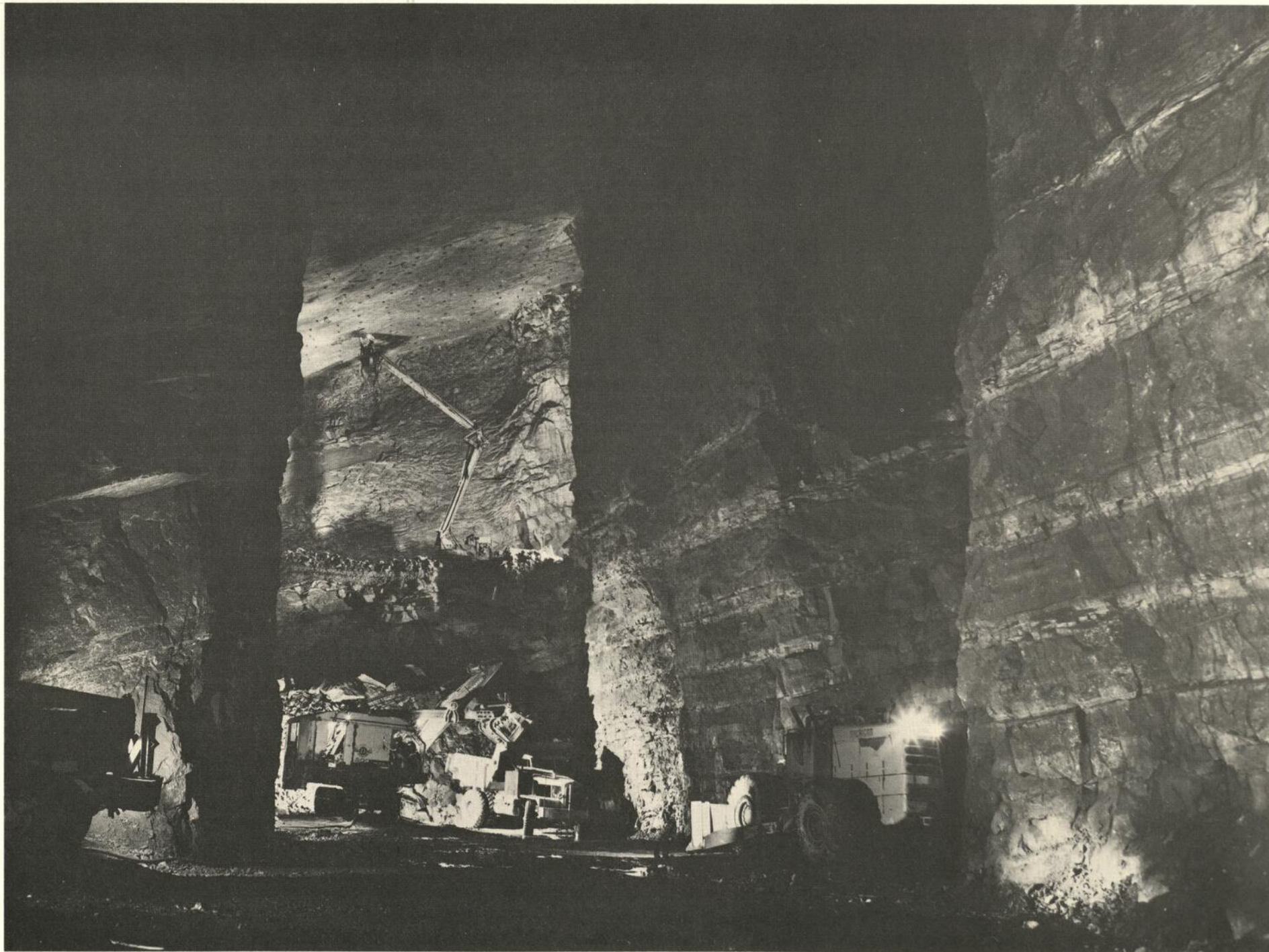
Underground showing "Giraffe" on roof bolting operations.
