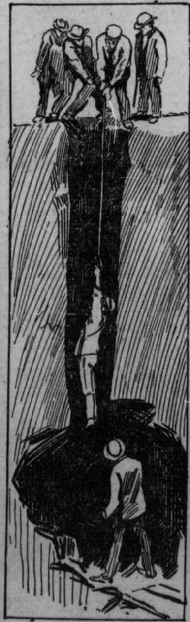
HOISTING KOSMELE OUT.
