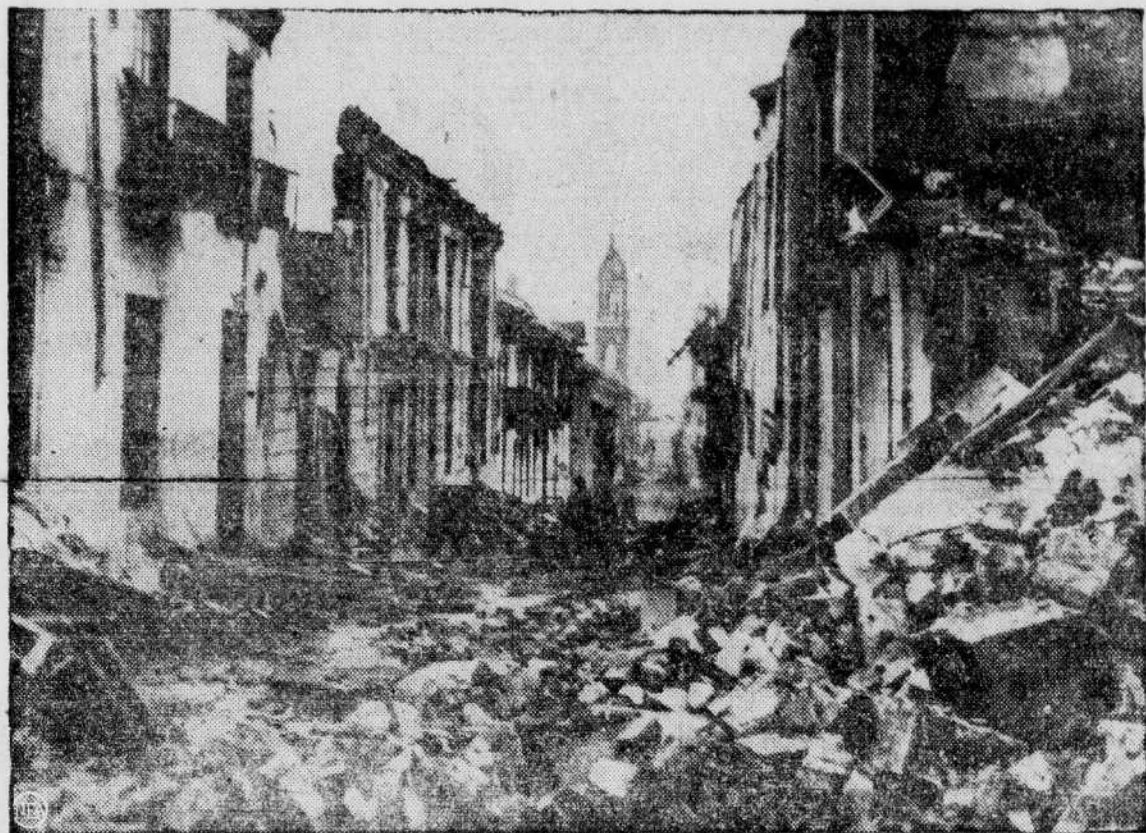
The warehouses and buildings on this street in Bogota were wrecked by rioters during the recent disturbances in the Colombian capital. The U. S. Export-Import bank has announced a credit of $10,000,000 to the Colombian government to help assist reconstruction of damage from last week's disorders.
