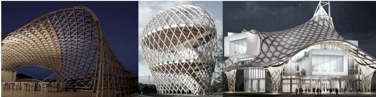
Figure 1 : Left : Toledo gridshell [I], Middle: Helsinki zoo, observatory tower (Paoli, 2007), Right: Centre Pompidou Metz (Lewis, 2011)
