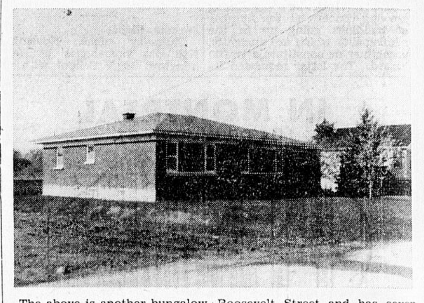
The above is another bungalow built by Earl Fournier Lumber and Construction Inc. for Mr. D. Leboeuf. This is situated on Roosevelt Street and has seven main rooms. It is the most recently completed.
