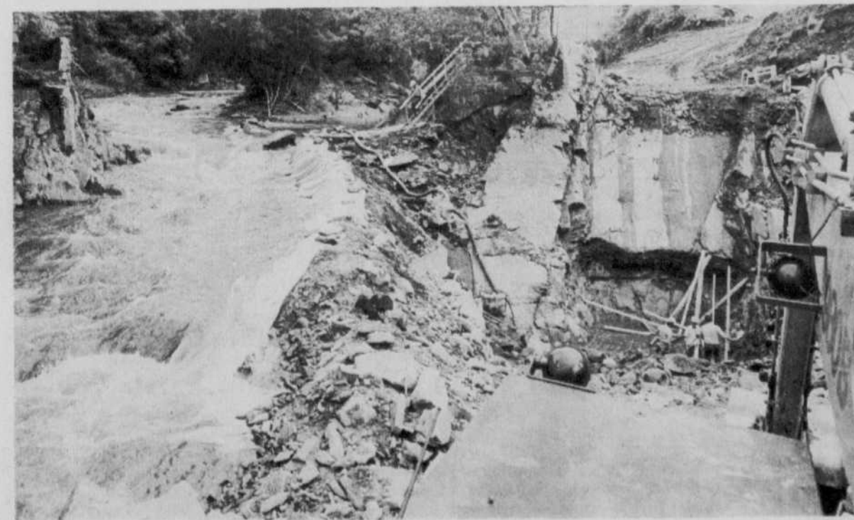
The river has been moved out of its bed so construction crews can build new dams and install new generators in Coaticook.
