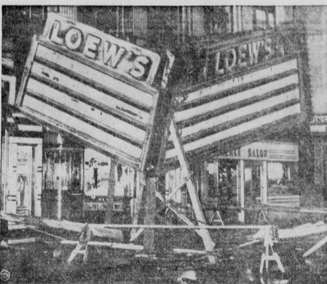
This theatre marquee at Indianapolis blew down as winds of 60 to 70 miles per hour ripped through the midwest. The marquee dropped to within five feet of the sidewalk. Workmen propped it up before it could do further damage.
