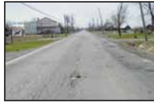
Figure 6 - RURAL - Route 235 Avant
