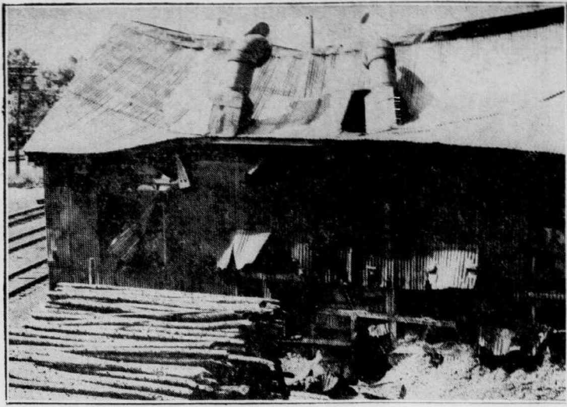
Twisted by the heat of flames, the Quebec Pipe Company plant in Lennoxville is pictured above following the fire which broke out on Tuesday, causing damages estimated at between $10,000 to $15,000. The fire there was the second within a week.
