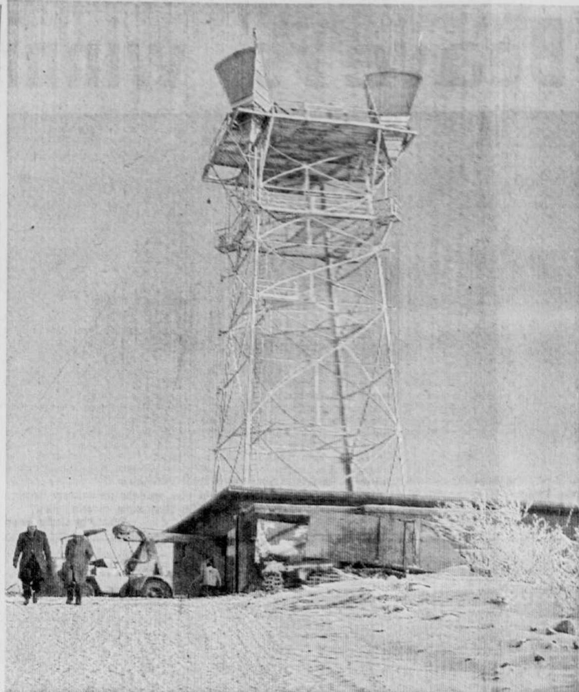
STATION-TOWER — Shown above is a new Bell Telephone microwave station-tower site at Foster Mountain, near Knowlton in the Eastern Townships. On top of the 100-foot tower are two of the giant horn antennae which provide transmission of long distance calls, commercial television programs and many forms of business communications throughout Bell's Quebec-Ontario microwave network. The Foster Mountain site is one of five station-tower sites on a new 207-mile route now under construction between Montreal, Sherbrooke and Quebec City. Other tower sites are at St. Alexandre, Sherbrooke, Stornoway and Tring Junction.
