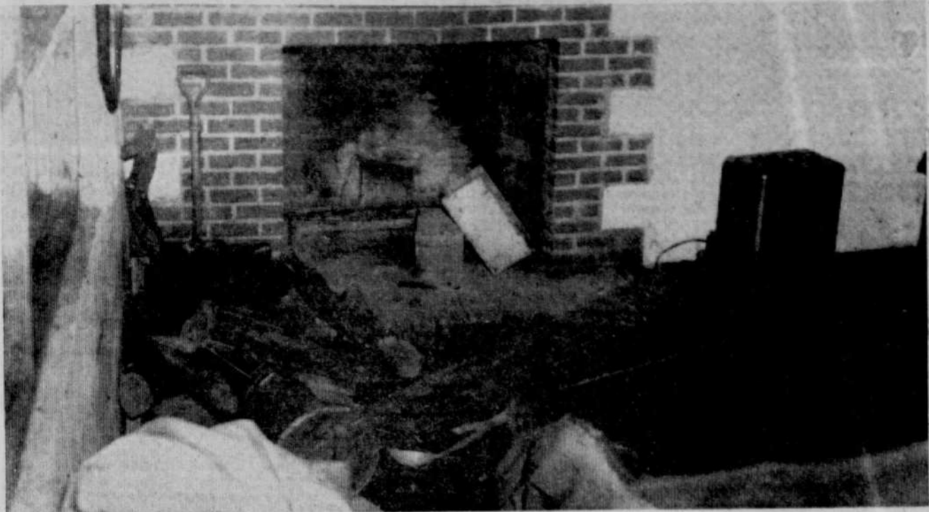
EXPLOSION DAMAGE — Wreckage covers the floor of the Rolnick cottage at New Boston, near Stanstead, following a propane gas explosion yesterday. Three people were burned in the flash fire that followed. (Record photo by Andre Pepin)
