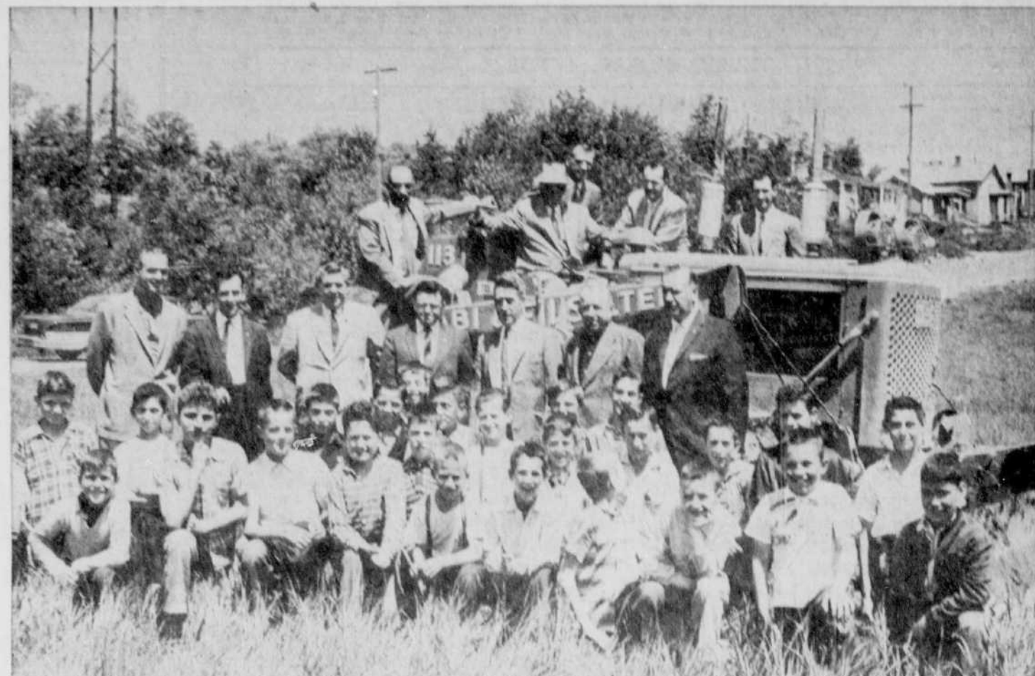
OPTIMIST POOL UNDERWAY — Ground was broken yesterday for the Sherbrooke Optimist Club swimming pool located in Assumption parish near the Pie X school. Work was gleefully supervised by a group of youngsters from the school. Pictured above with the youngsters are Optimist Club and civic officials. Seated on the bulldozer, from left to right: Angelo Fabi, president of Fabi et Fils, Ald. J. M. Jeanson, Gene Marcoux and Club President Art Lockley. Standing, from the left: Leon Beaudry, Pierre Rochette, Claude Genest, Henry Crocheteire, Ald. Robert Gauthier, Erich Marquardt and Ivan Dugre. (Record Photo by Gerry Lemay)
