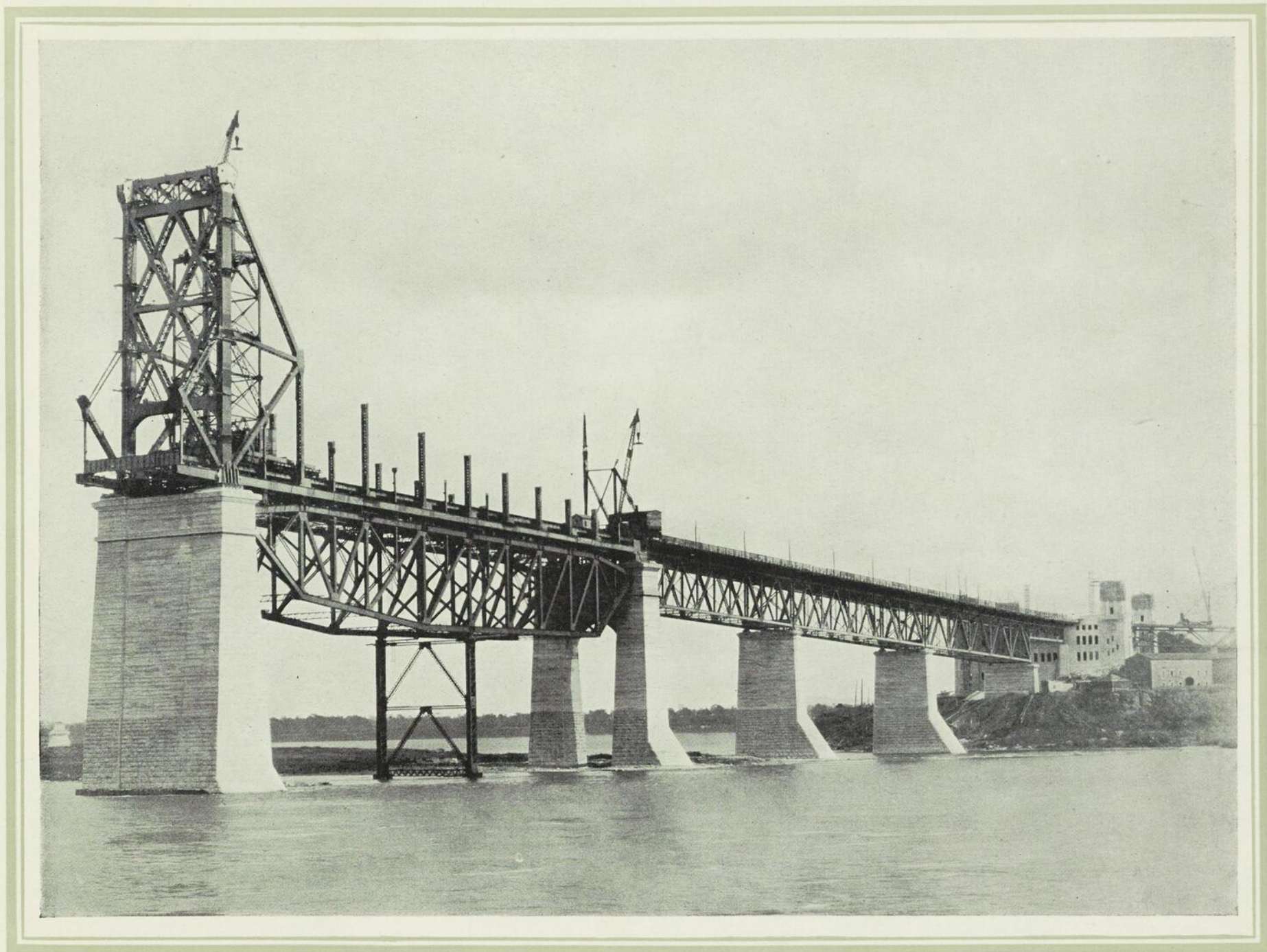
Figure 23. —ERECTION PROCEEDING ON SOUTH ANCHOR ARM.
