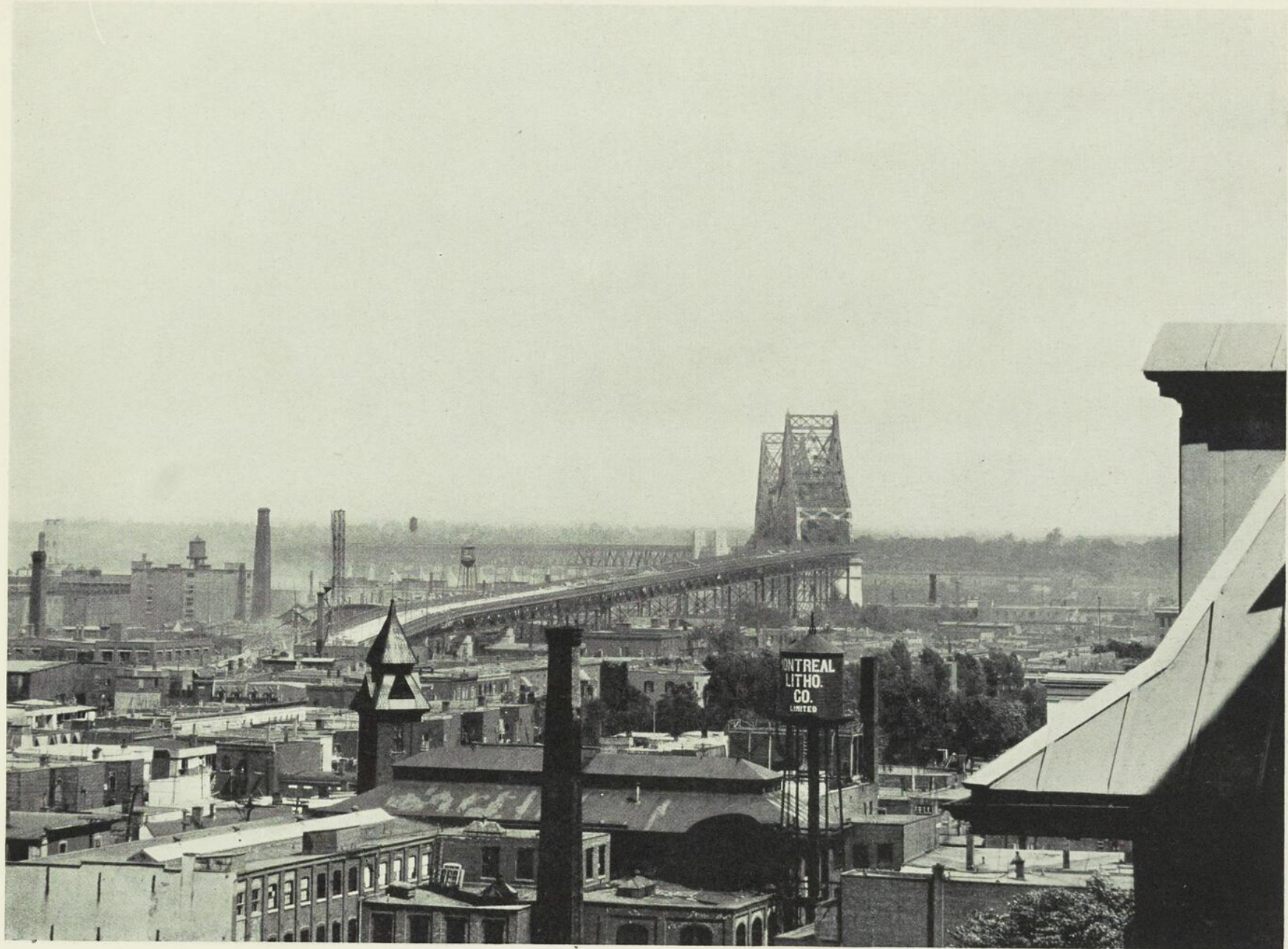
Figure 35. —THE BRIDGE AS SEEN FROM THE MONTREAL END.
