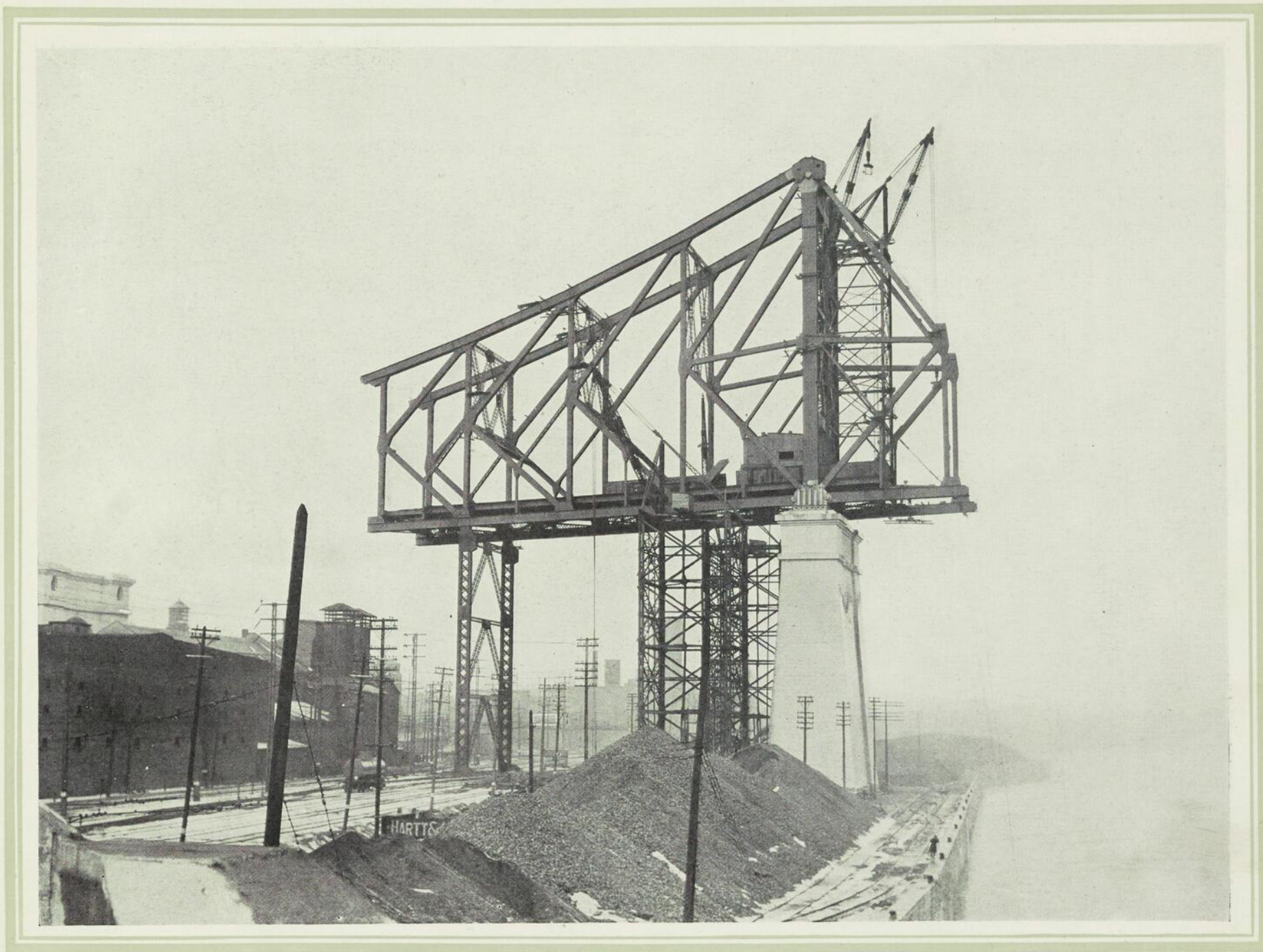
Figure 13. —PROGRESS ON NORTH HALF OF MAIN SPAN AT DECEMBER 14TH, 1927.
