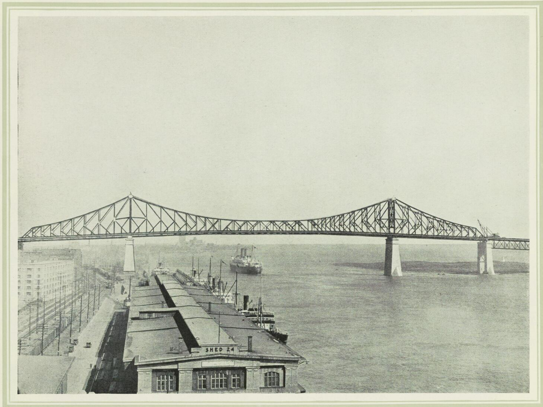
Figure 34. —ERECTION OF MAIN SPAN COMPLETED, FALSEWORK REMOVED, AND EQUIPMENT BEING DISMANTLED. S.S. "DUCHESS OF ATHOL" IS SEEN PASSING UNDER SPAN.
