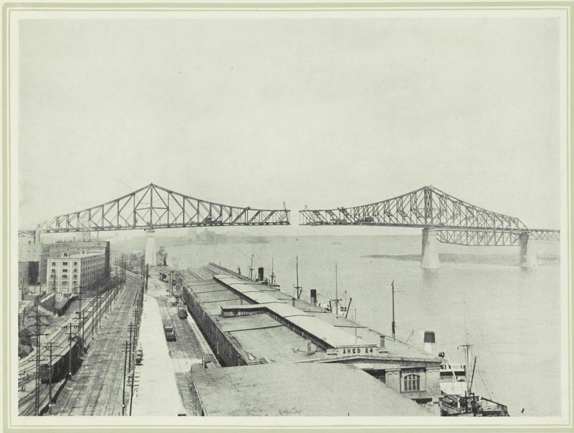
Figure 27. —PROGRESS ON MAIN SPAN AT JULY 1ST, 1929.
