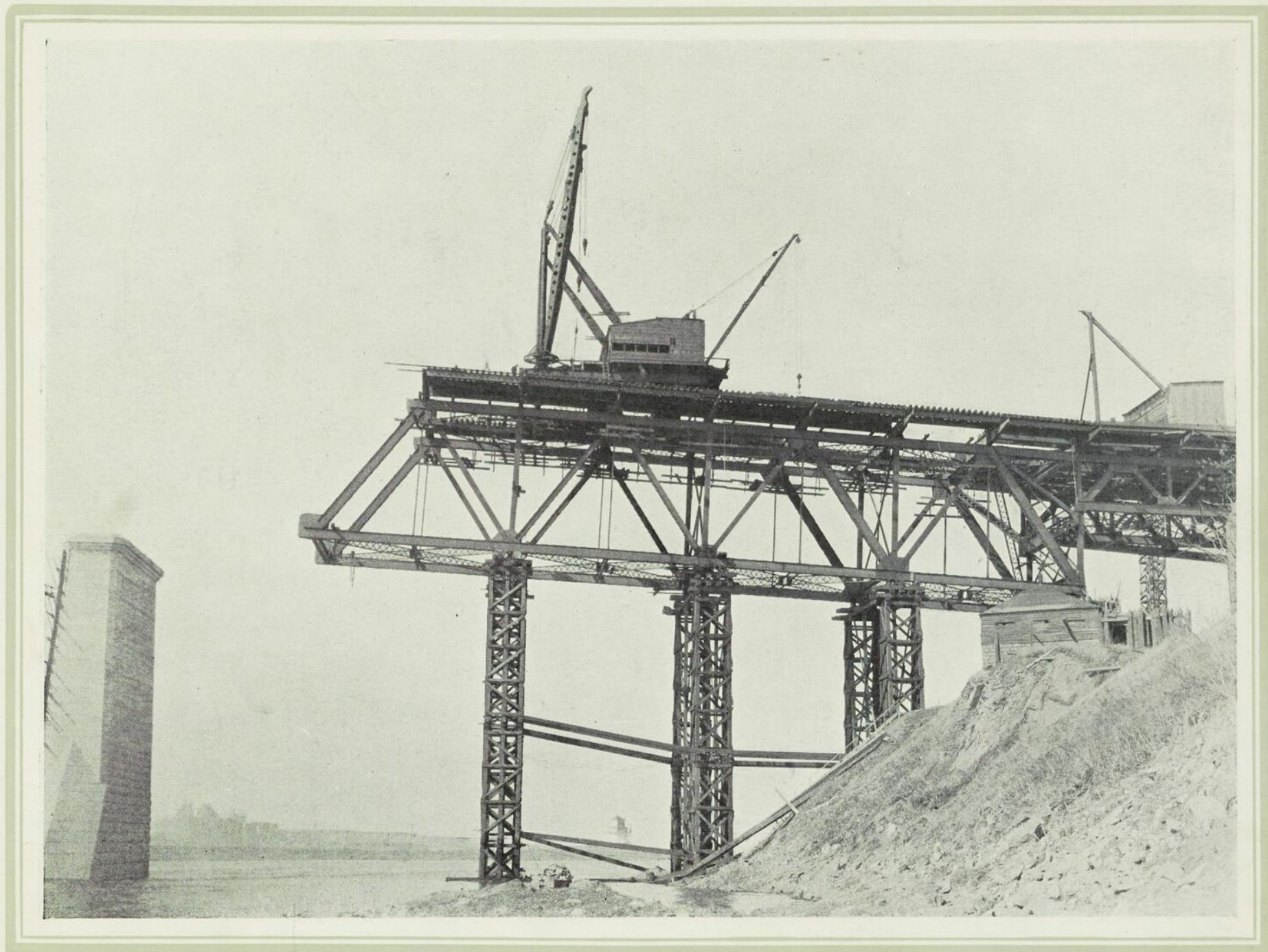
Figure 9.—ERECTING FIRST 245 FOOT SPAN NORTH OF PAVILION.
