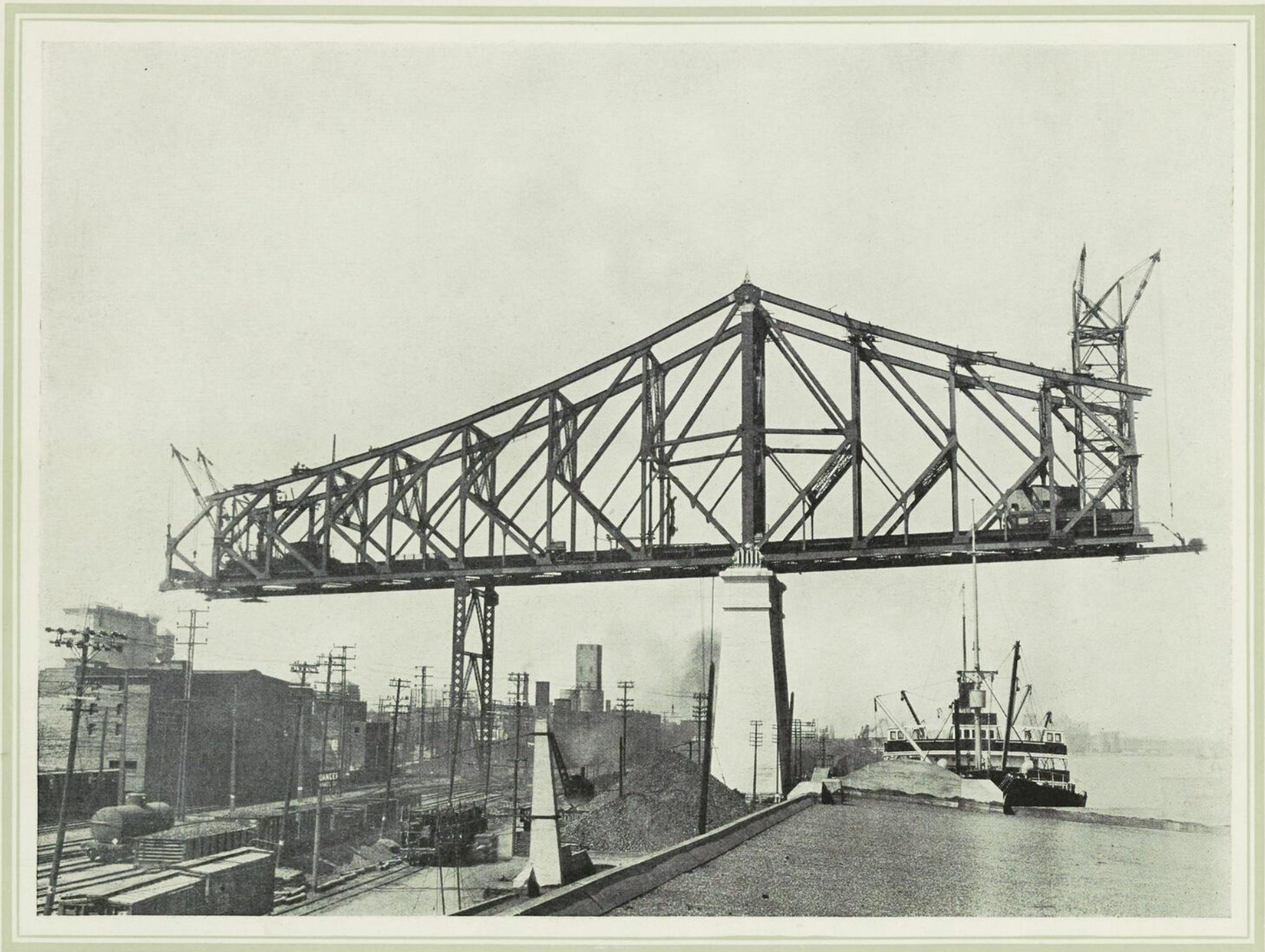
Figure 14. —CONCURRENT ERECTION OF NORTH ANCHOR AND CANTILEVER ARMS.
