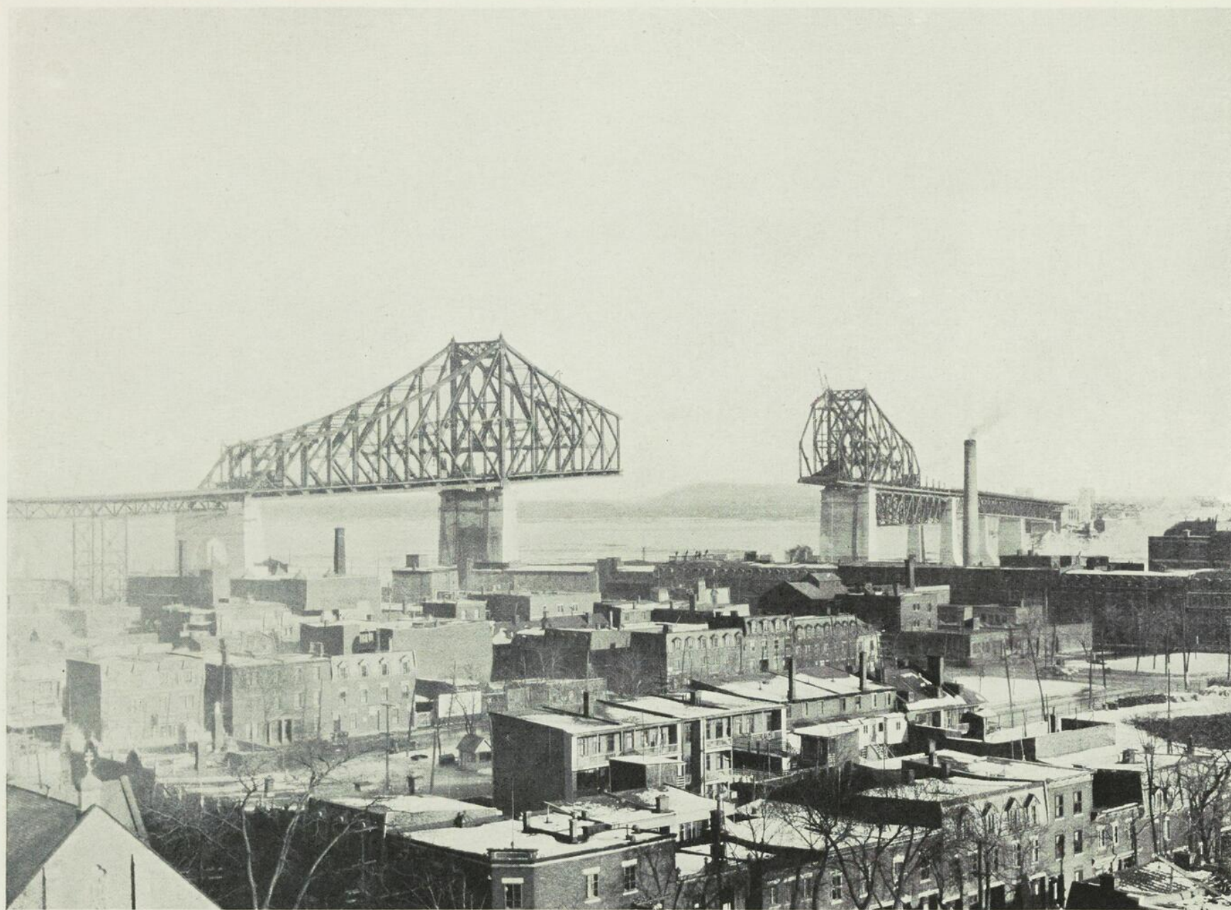
Figure 24.—PROGRESS ON MAIN SPAN AT DECEMBER 14TH, 1928.
