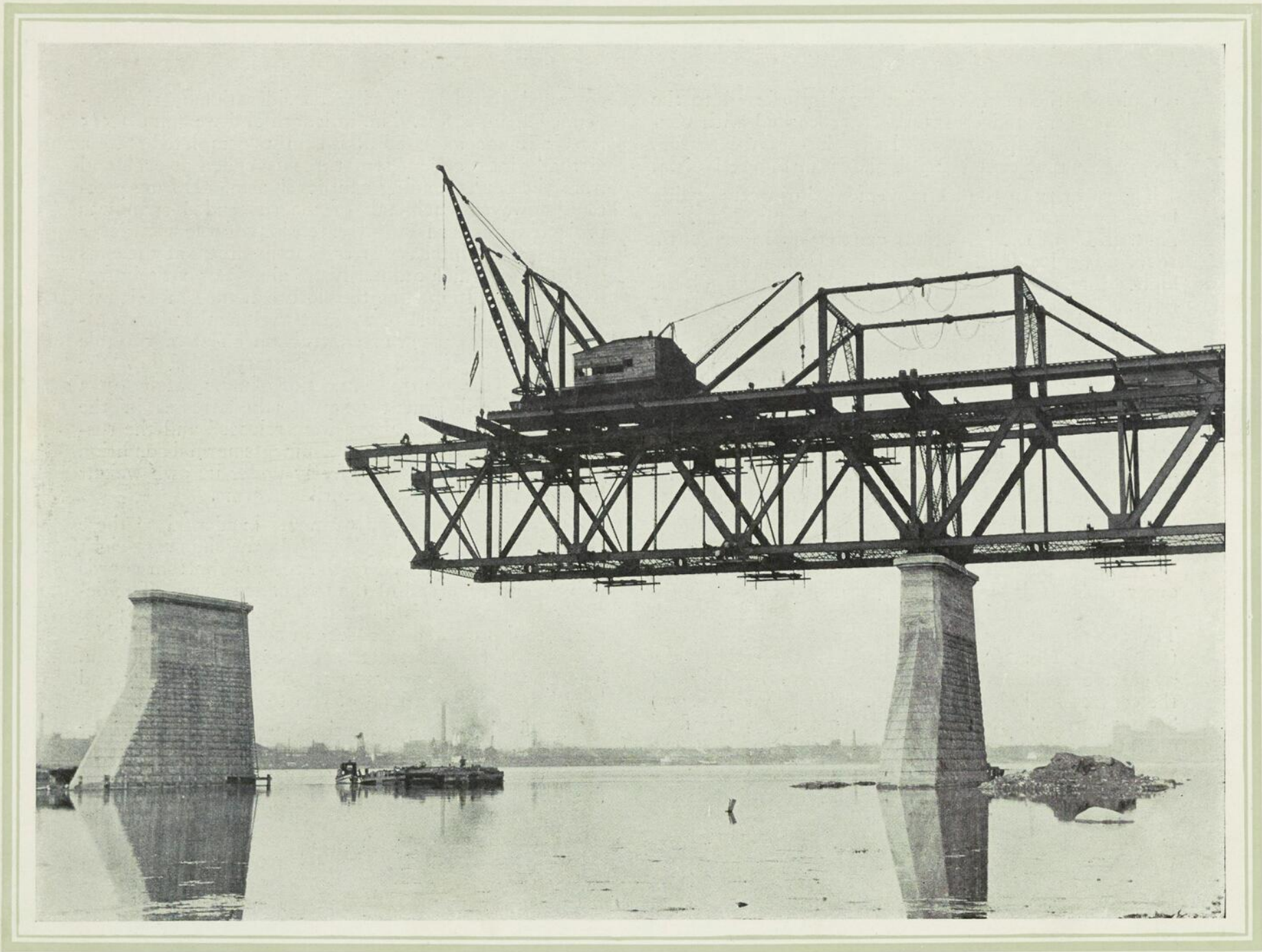
Figure 8.—CANTILEVER ERECTION OF 245 FOOT SPAN OF SOUTH APPROACH.
