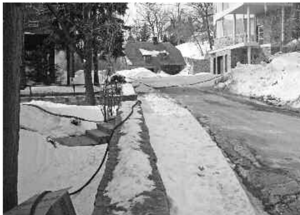
A temporary hose feeding up from a fire hydrant on Belvedere at The Boulevard was still being used March 20 as a temporary source of water for two houses on either side of Trafalgar Ave.
