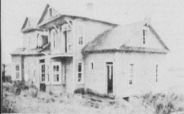
Abandoned Hotel, St. Jacques de Leeds
