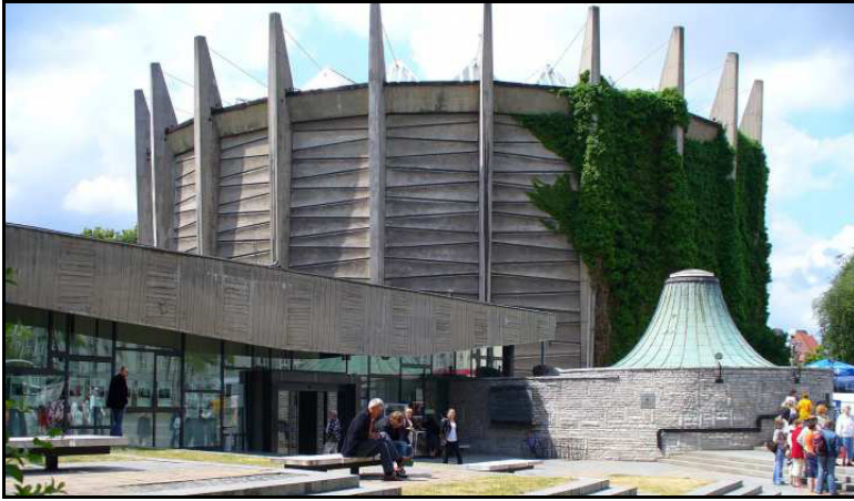
Figure 5.50: Panorama Raclawicka building.
