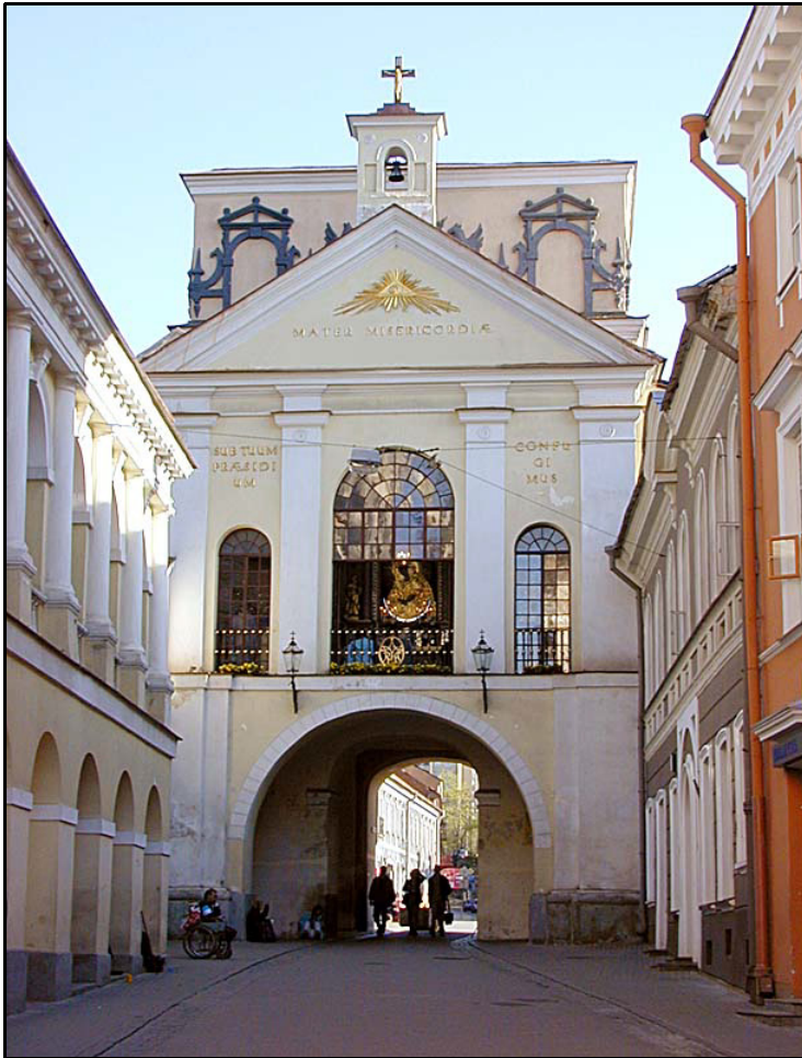
Figure 3.6: City gate from inside.
