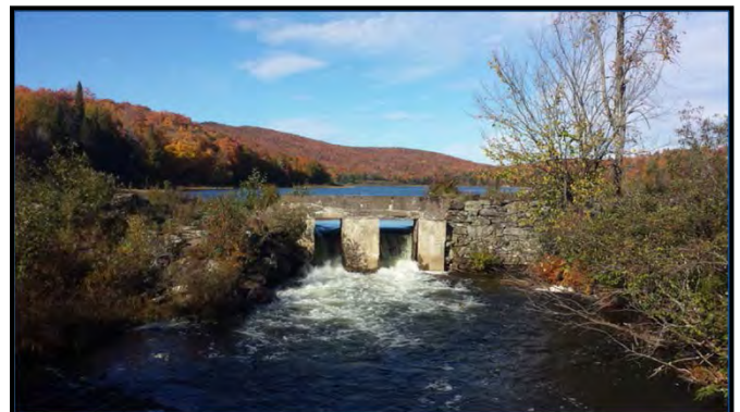
The Fullerton Pond and dam David Brisson | 2016
