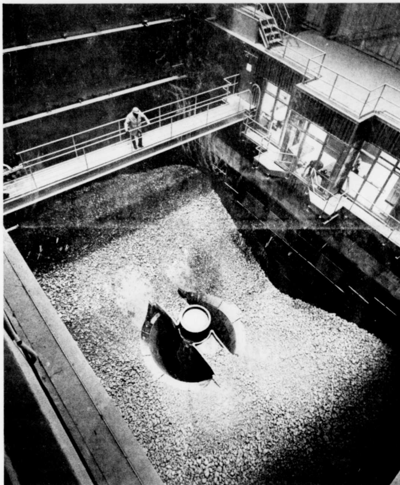
THE CRUSHER — What is believed to be the biggest ore crusher in the world has entered production in the new Canadian Johns-Manville crusher-dryer-concentrator complex in Asbestos, part of the company's $75 million, three-year program to relocate surface facilities at the Jeffrey Mine. Trucks of up to 200 tons capacity will dump as much as 3,000 tons of ore hourly into the manganese-steel-lined crusher pit, filled with rock at a
