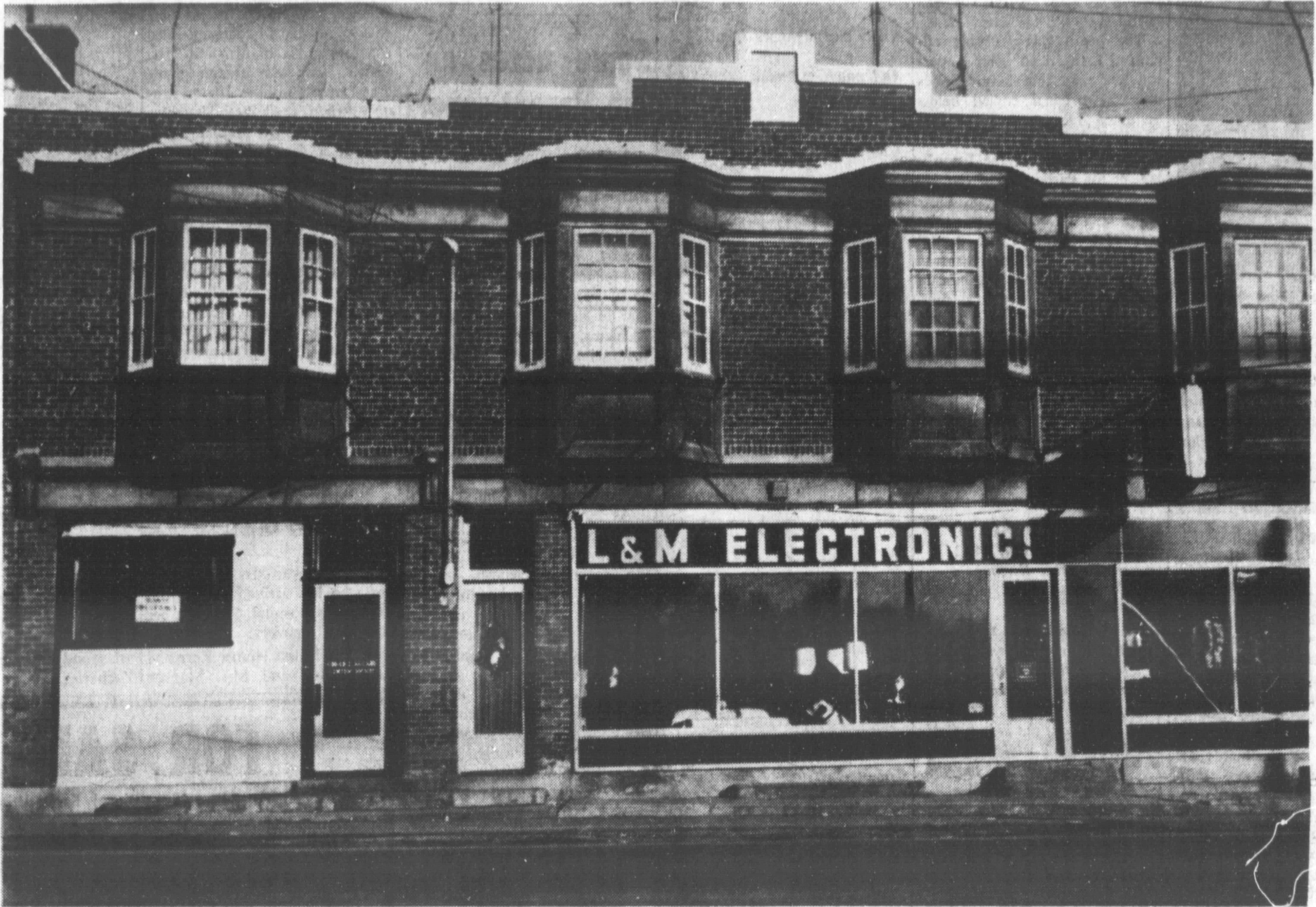
The Hanrahan building situated on Main St. of Campbell's Bay, was SOLD by ANDRE AUDET agent for ANDRE TESSIER Limited Real Estate, Hull —Audet Studio Photo
