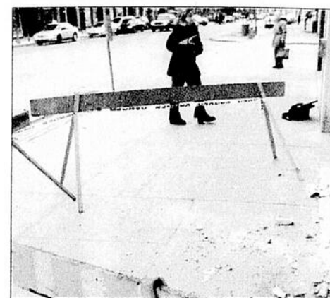
Barriers were still in place last week to keep pedestrians from being struck by debris falling off the front of a three-storey Sherbrooke Street building.
