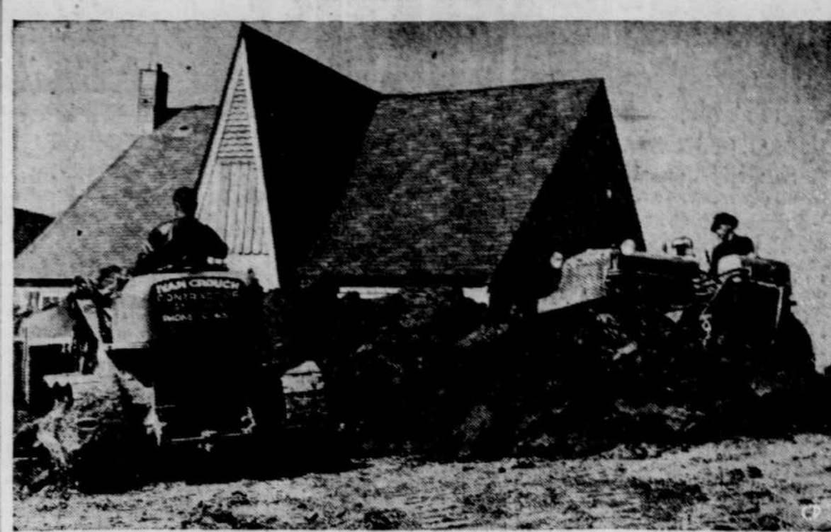
The Lyndale Dike, which held back flood waters on the Red River from Norwood homes, is being removed. Here bulldozers chew away the great pile of rubble which once was the homes it surrounded. Removal of the dike was urged by residents of St. Boniface, anxious to return to their homes.
