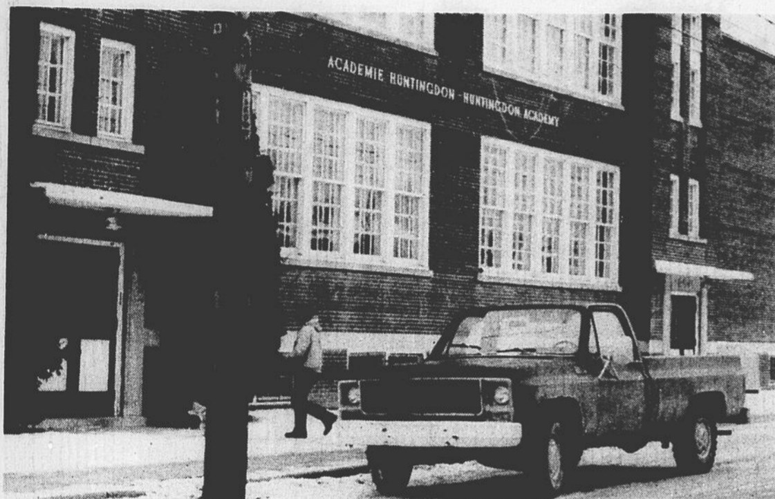
Huntingdon Academy will get a new roof, with the aid of a government grant.
