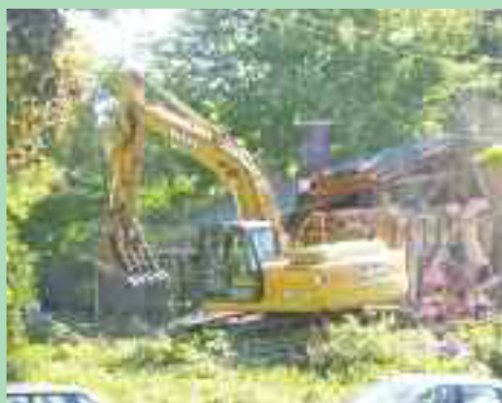
Flattened: 31 Willow Ave., p. 23 photo: Carol Kremer.
