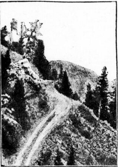
Improved Road in Oregon.
