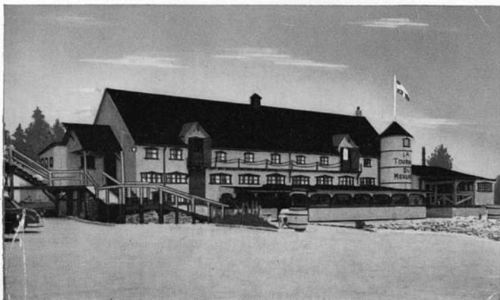
"LA TOURNÉE DU MOULIN", AN UNUSUAL BARN LIKE A RESTAURANT. CHARLESBOURG, QUE., ON ROUTE 54.
