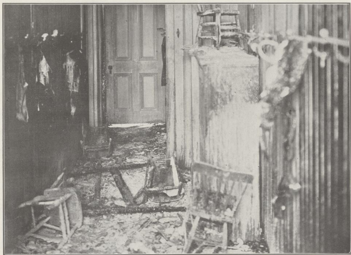
INTERIOR OF THE HOHELAGA FIRE TRAP—The dressing-room, adjoining the kindergarten classroom, to which some of the doomed children ran when the alarm of fire was given. Near the window there is evidence that the flames had a fierce innings for a brief time, but towards the door which opens into the corridor they had hardly any sweep at all, and some of the coats hanging on the pegs in the illustration are absolutely unharmed. The first thought of the children was to save their clothing, hence the fatalities in this part of school.
