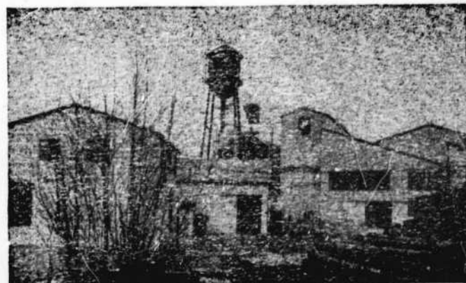
Siscoe Milling Plant, showing mill feed, bucket on the aerial tramway. Length of tramway 800 feet.
