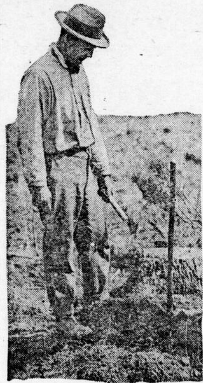
GETTING READY TO BLOW UP A STUMP.
