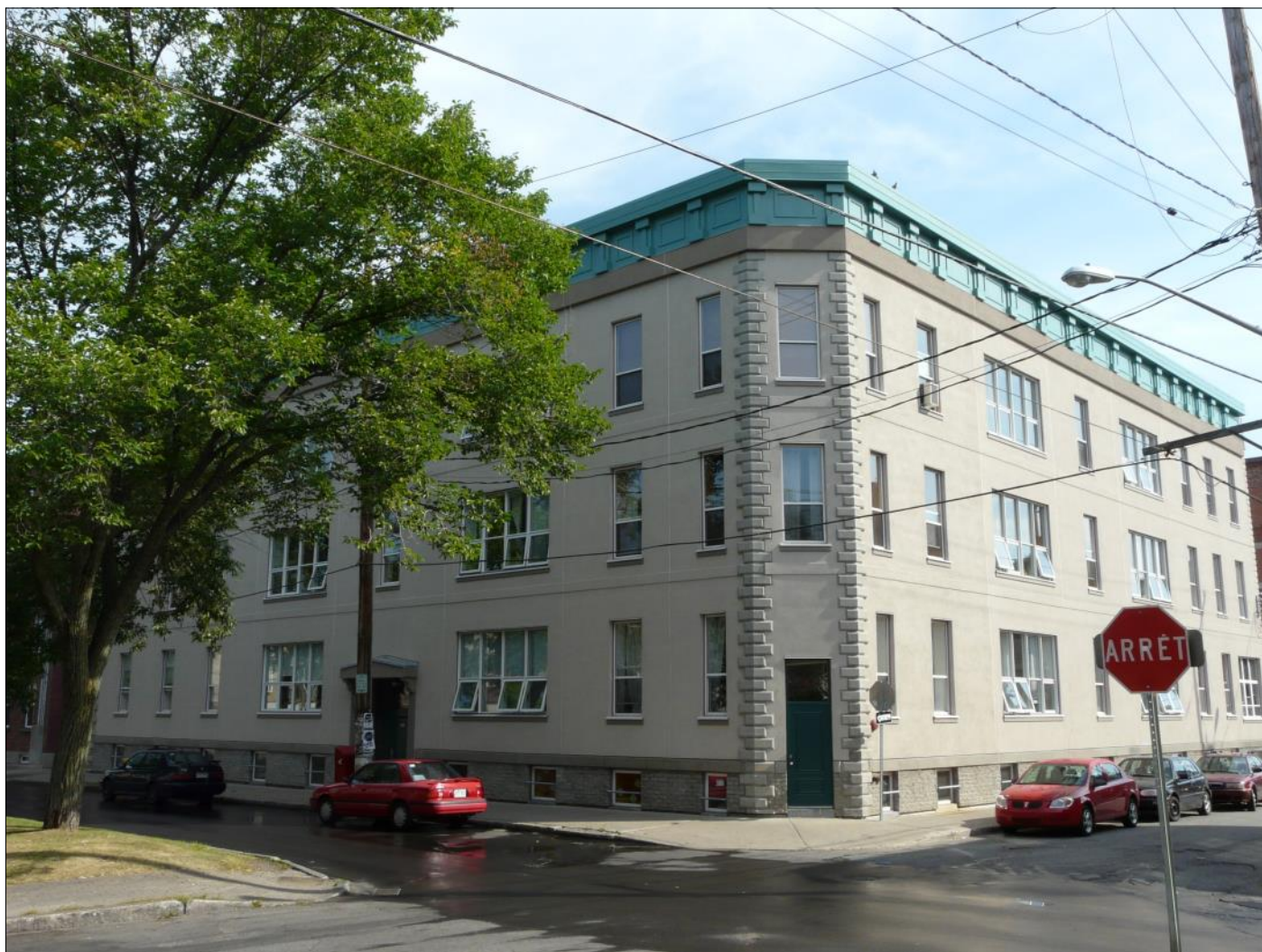
The Royal Paper Box Co. was built in 1908 at the corner of Langelier and Christophe Colomb Streets in Quebec City. It is now a condominium building. (Photo: Quebec City, 2008)
