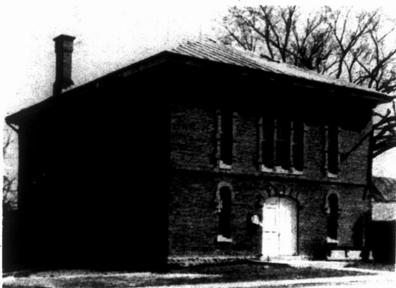
The former Hemmingford Town Hall which is now demolished.
