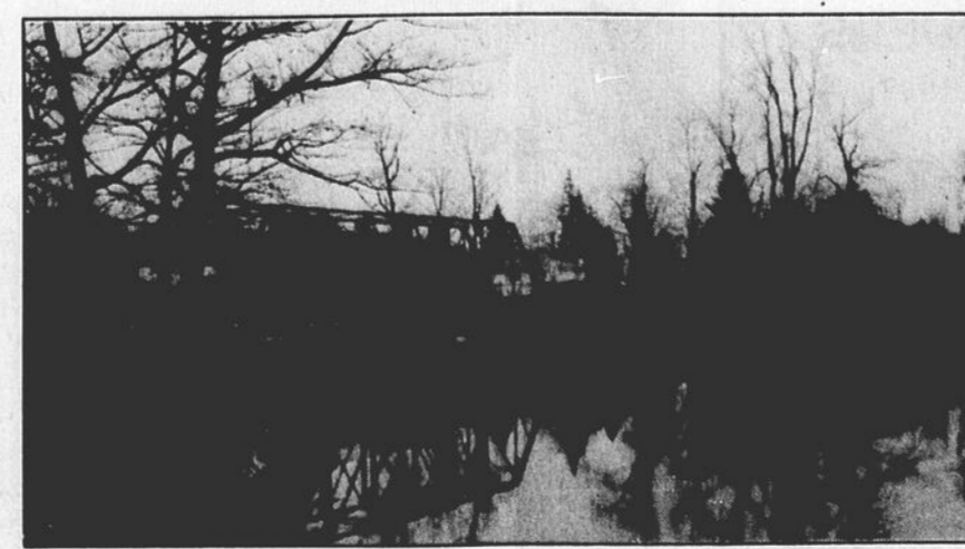
Looking downriver toward the Dewittville bridge.
