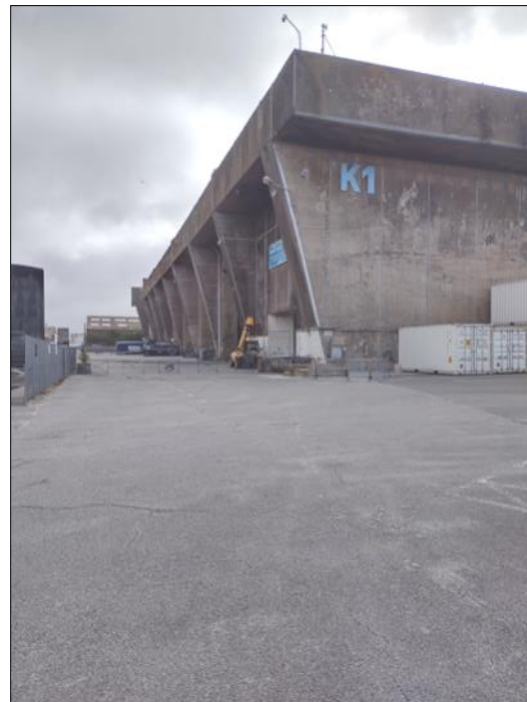
Bunker Keroman 1 in Lorient (Photo: André Kirouac)
