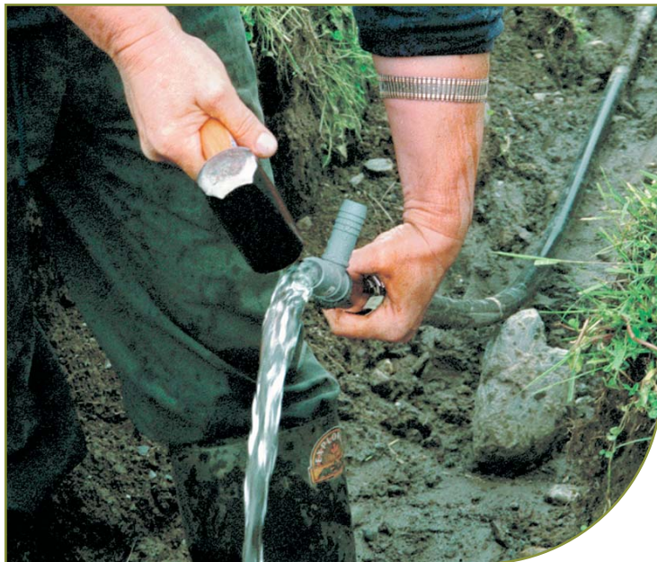
USE 100-PSI PIPES OF THE RIGHT DIAMETER.
