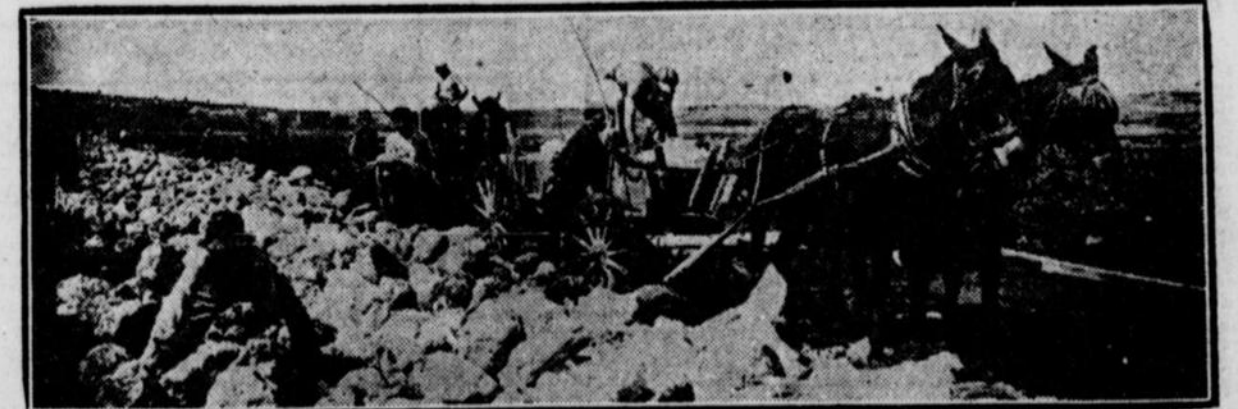
The return of many Jews to the Holy Land has resulted in modern ideas being put into practical use. Roadbuilders are shown unloading stones for the construction of an up-to-date highway
