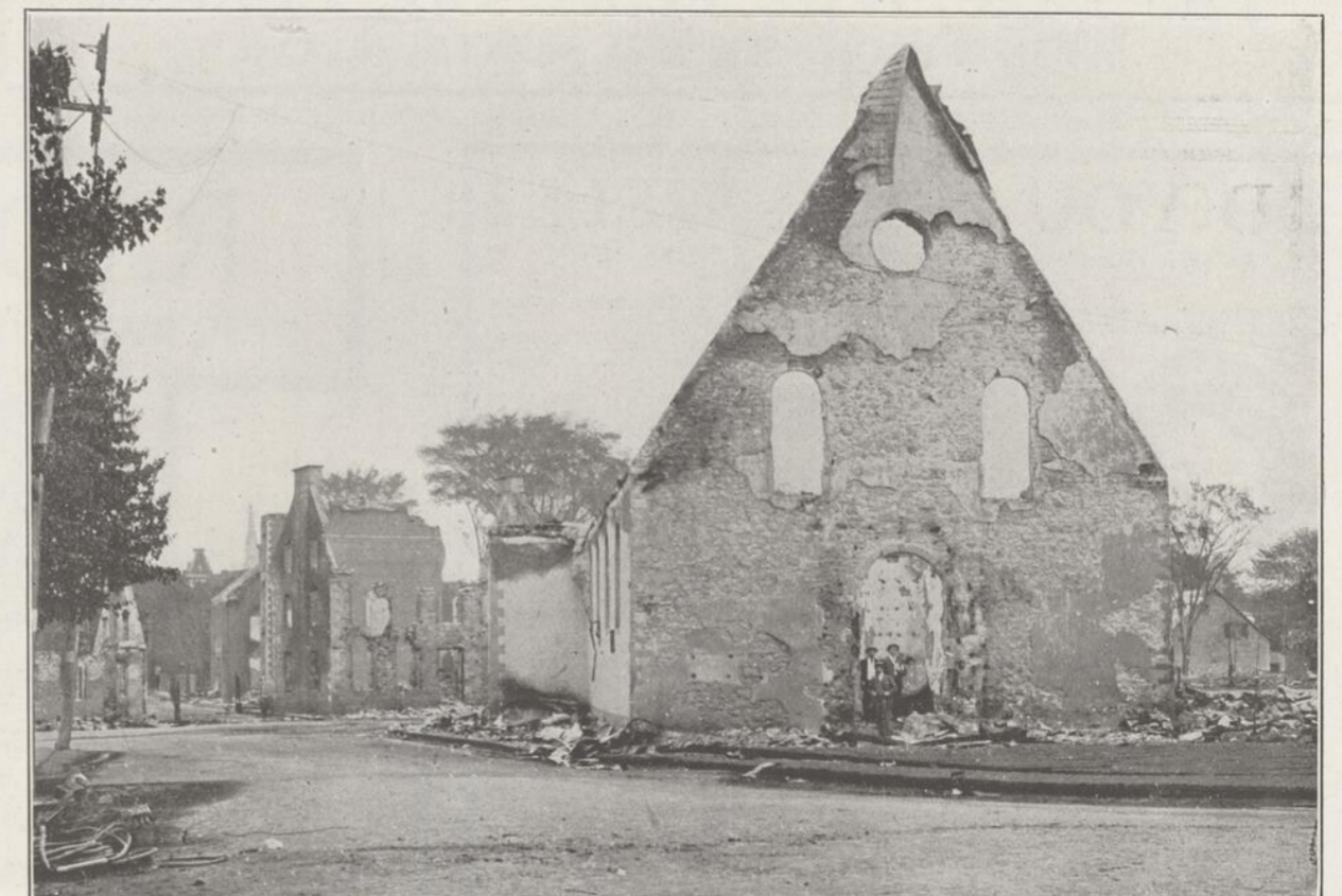
THE RECENT CONFLAGRATION AT THREE RIVERS—All that remained of the Roman Catholic parish church on the morning after the fire. This edifice was one of the oldest and most historic edifices in Canada, and its destruction is greatly deplored. It had been in constant use since the middle of the 17th century, and was a link connecting the present materialistic century with the chivalrous days of the old French regime. It is a unique Canadian landmark, and a building that could ill be spared.
