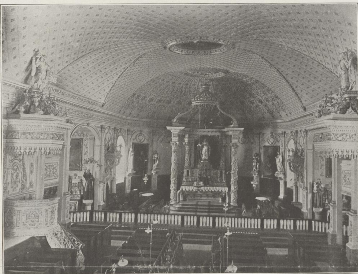
THE RECENT CONFLAGRATION AT THREE RIVERS—Interior of the Parish Church, which was completely gutted by the flames. This edifice was one of the oldest churches in Canada. It was originally built in 1664, but was re-constructed in 1714, since which time few changes have been made in its appointments.
