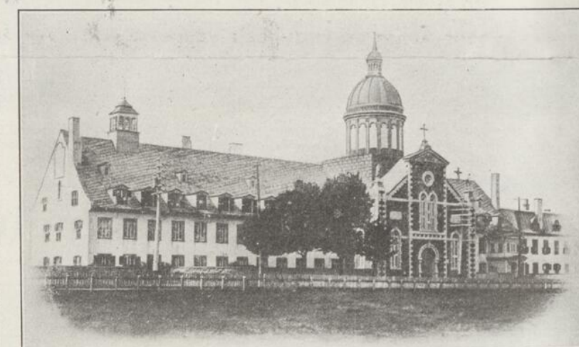
THE RECENT CONFLAGRATION AT THREE RIVERS—Exterior of the Ursuline Convent, one of the oldest community houses in Canada. This building was frequently attacked by the flames, but the firemen succeeded in saving it from destruction.
