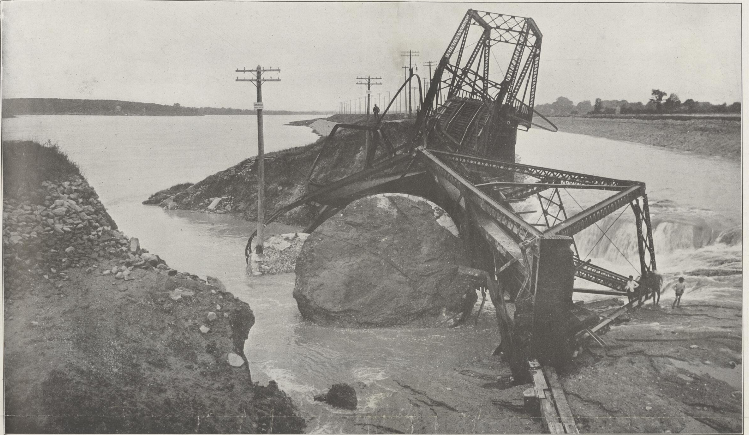
THE BRIDGE COLLAPSE ON THE CORNWALL CANAL—The above illustration shows the immense damage caused by the recent break in the embankment separating the waters of the Cornwall Canal from those of the St. Lawrence, near Cornwall, Ont. Not only was the canal rendered useless for several weeks to come by the accident, but the swing bridge of the Ontario & New York Railway was totally wrecked. The illustration shows the ruins of the bridge, the overturned pivot pier, the bed of the drained canal and the immense hole that the rushing waters caused in the canal bank. The damage to the canal is now being repaired, upwards of 200 men being at work on the construction of a new channel.
