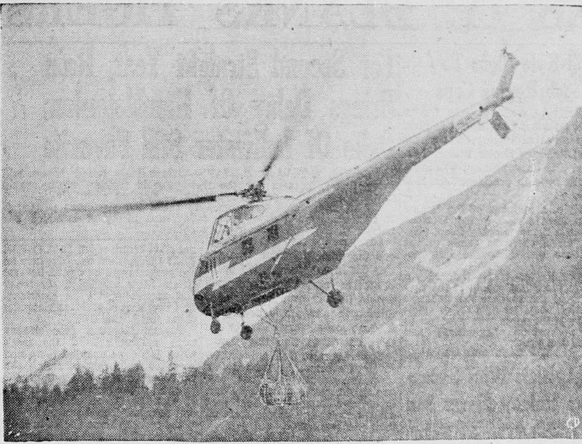
KITIMAT AIRLIFT —Eagles and helicopters share Kildala Pass where a power transmission line is being built for the world's largest aluminum smelter at Kitimat, B.C., 450 miles north of Vancouver. Construction camp 11, which is 5,300 feet above sea level and 2,000 feet above timber level, has all its supplies brought in by helicopter, some machines making 25 and 30 trips daily. Kildala Pass summit is the loftiest summit on the 50-mile transmission line. The pass section covers 10 1/2 dizzy miles. (CP Photo)
