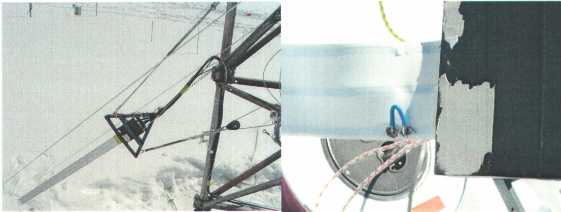
Figure 9 - Installed cable at Swiss test site and repair of broken conductor
