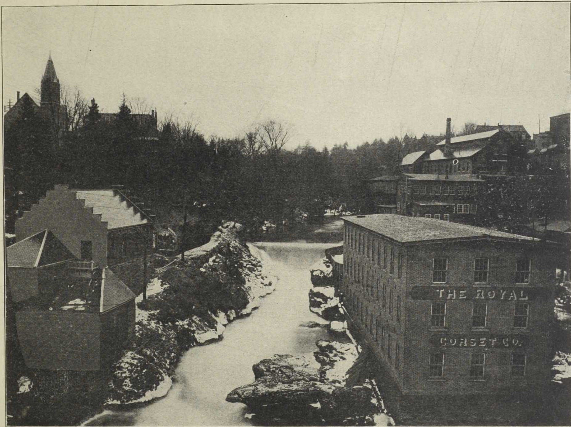
VIEW OF WATER POWER (DAM No. 4) MAGOG RIVER.
